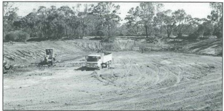
Cleaning of Yornaning Dam.
