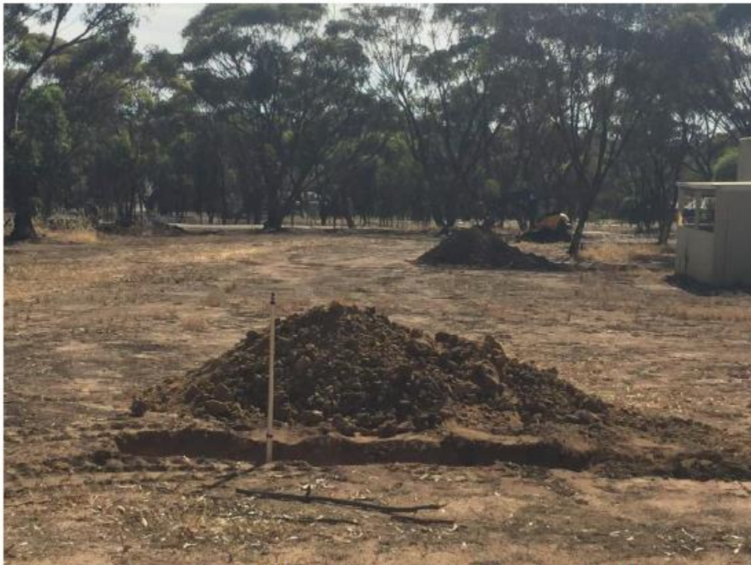
Site Photo showing testholes across Lot 8 – Testhole #1 is in the foreground. Note the 8T Mini Excavator in the background.
