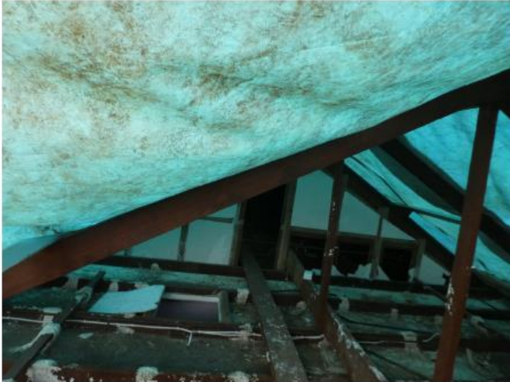
Figure 13; The Props Need to be Fixed to the Ridge Beam and to the Hanger Beam with 25x1mm Galvanised Strapping each side and Tek screws or two 10mm bolts.
