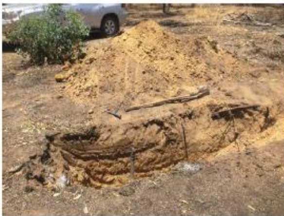
Testhole #5 – with excavated material
