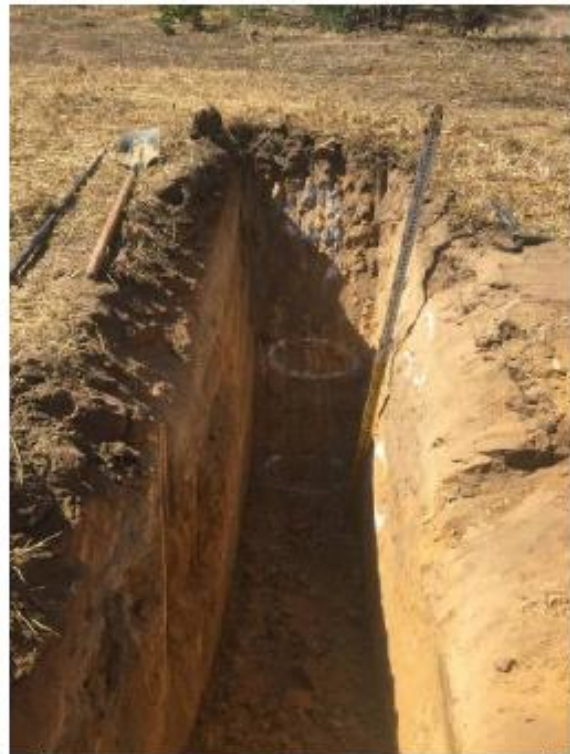
Testhole #9 - with number marking.
