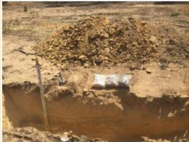
Soil Sample bags 7A, 7B & 7C on ground above Testhole #7.
