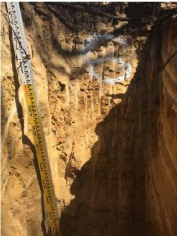
Testhole #6 – showing sample excavation locations.
