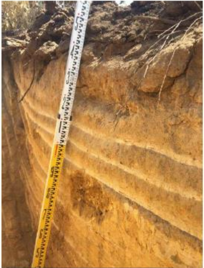
Testhole #6 – showing sample excavation locations.
