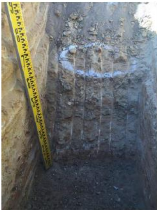
Testhole #9 – showing sample excavation locations.
