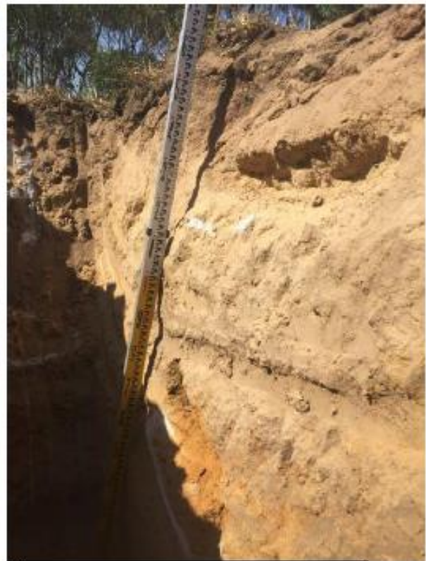
Testhole #9 – showing sample excavation locations.
