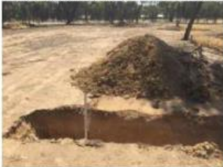
Testhole #2 – with excavated material
