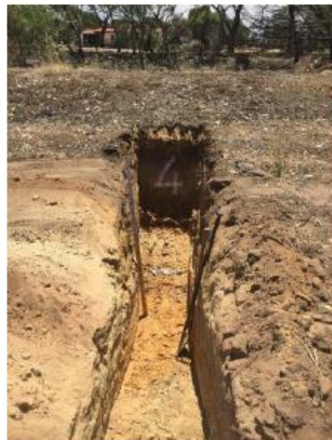
Testhole #4 - with number marking.
