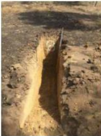
Testhole #8 – with number marking.
