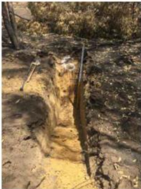
Testhole #6 – with number marking.
