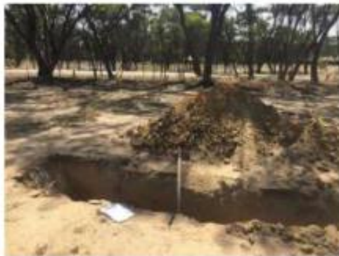
Testhole #3 – with excavated material
