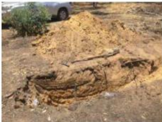
Testhole #5 – with excavated material
