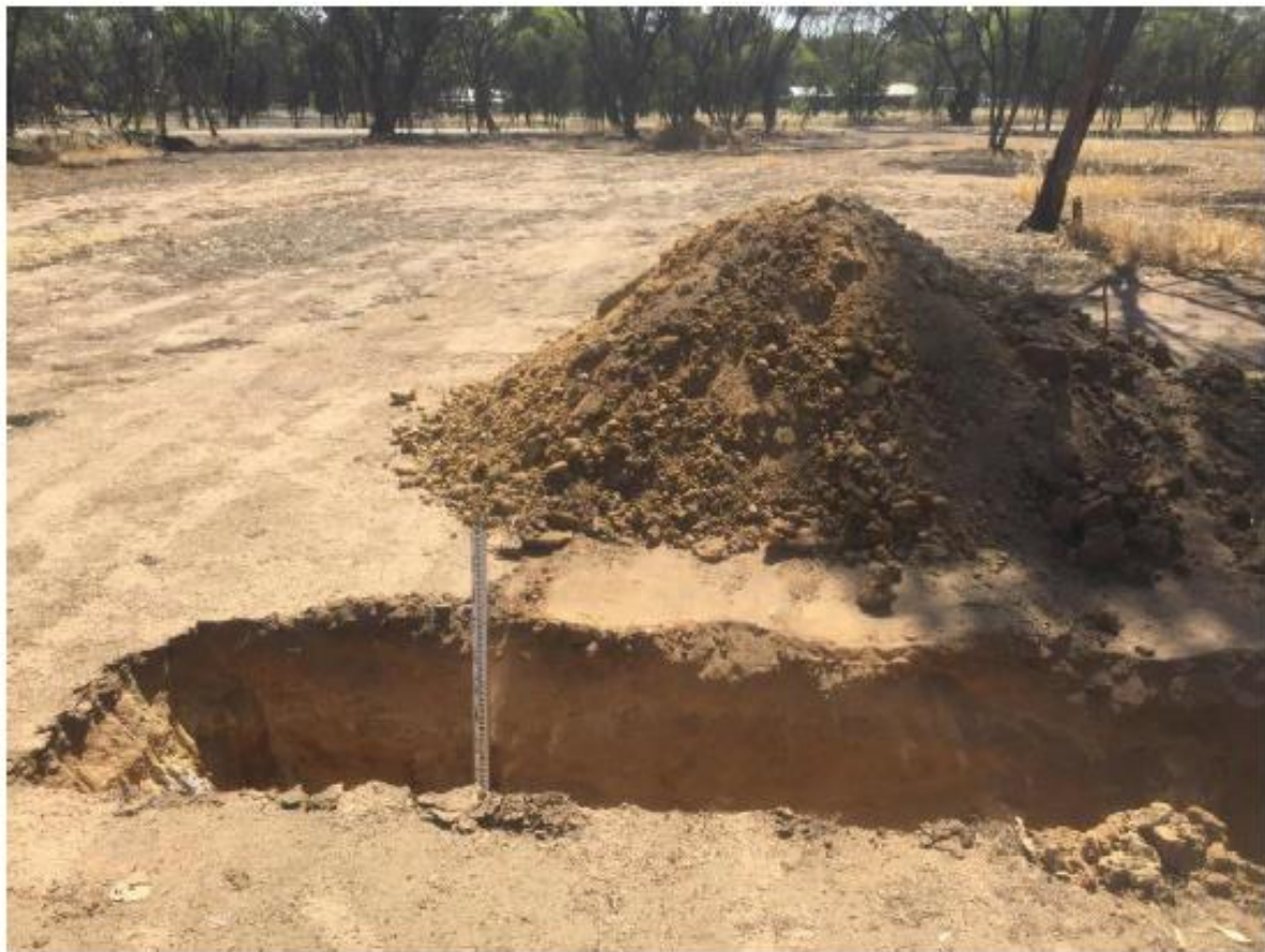
Testhole #2 – with excavated material
