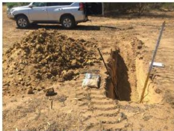
Soil Sample bags 1A & 1B on ground above Testhole #1.
