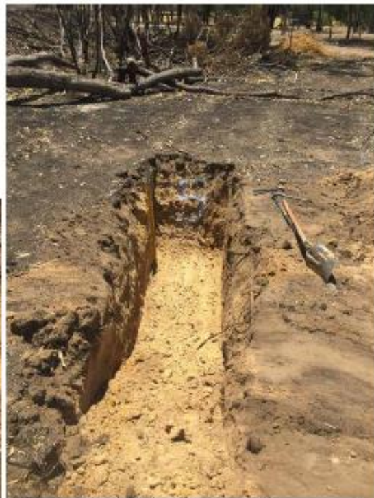
Testhole #5 – with number marking.
