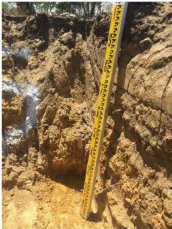
Testhole #5 – showing sample excavation locations.
