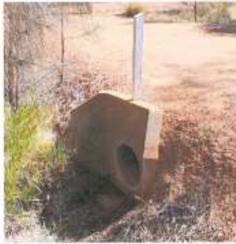
Eastern end of the culvert showing the concrete headwall and compacted gravel
