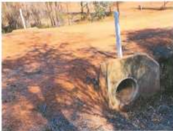
Western end of the culvert showing the concrete headwall over the end of the pipe and the white marker post
