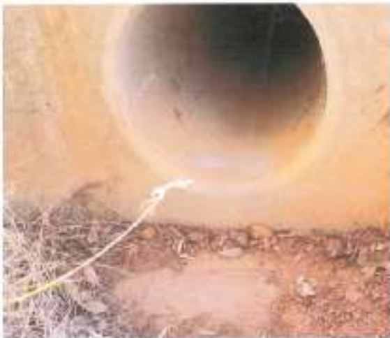
Eastern end of the culvert showing the concrete footing at the base of the pipe
