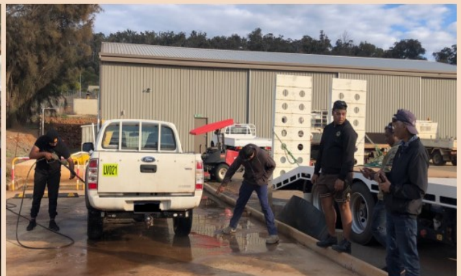
Vehicle wash down to remove soil and weed seeds
