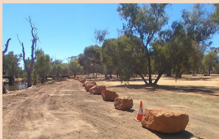
Image: River bank protection at Pumphreys Bridge
