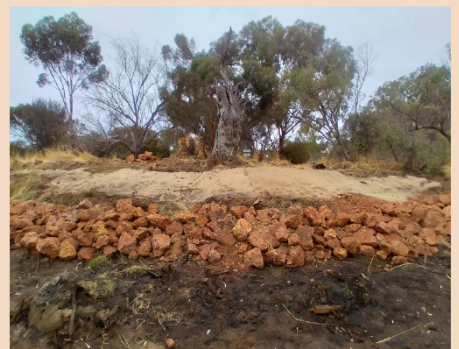
Image: Williams bank stabilisation (Planting on river bank to occur in winter)
