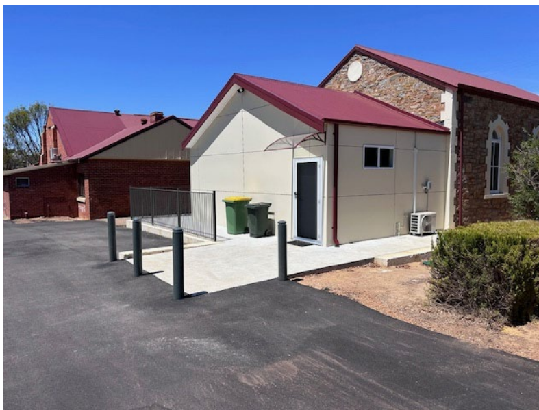
The upgraded CWA Hall
