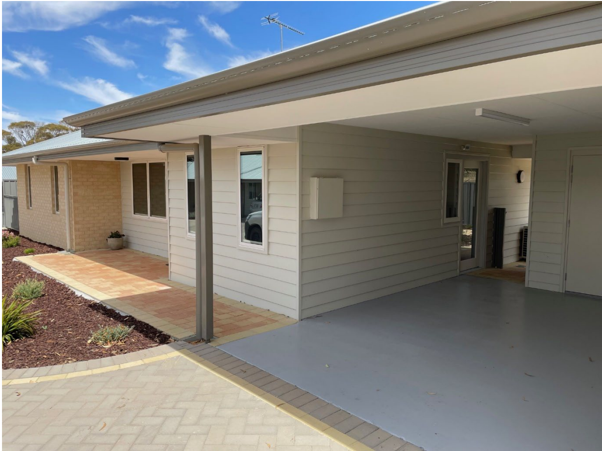
One of the completed units
